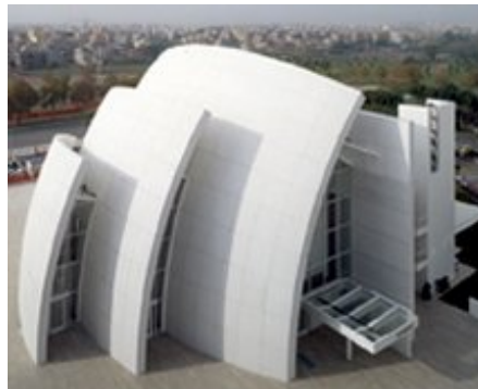
SACRED SURFACES. The modern church Dives in Misericordia located in Rome, is made from a self-cleaning concrete that breaks down atmospheric pollutants that would otherwise darken the surface over time.
