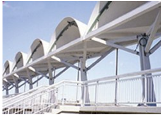
FACING THE FUTURE. A light-rail transit station in Calgary, Alberta, (above) and face sculptures adorning a condominium complex in Vancouver, British Columbia, (below) are made from new high-tech concrete materials.
